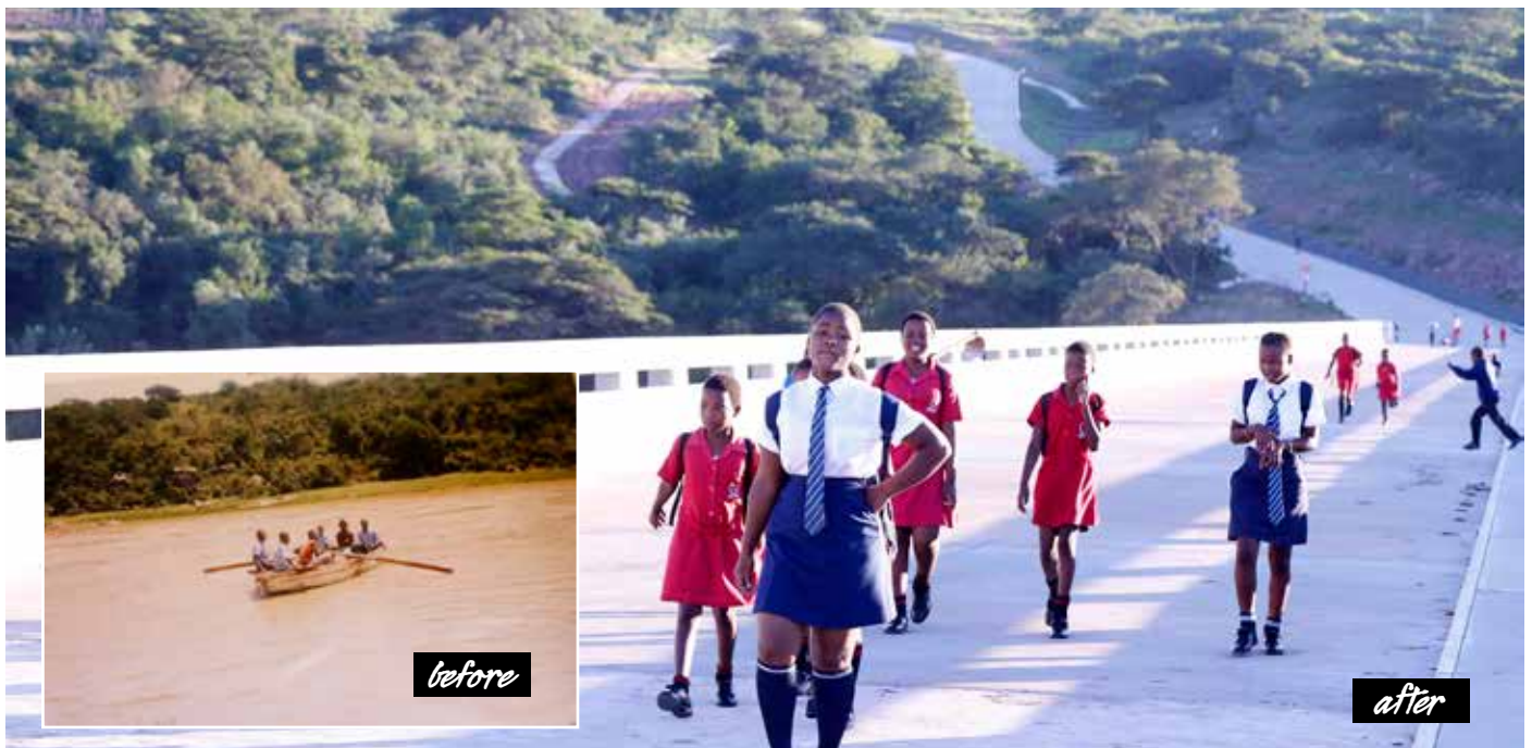
The inserted picture shows learners crossing Uthukela River using a boat. The main picture shows learners walking on the newly built Nyakana Uthukela River Bridge, which connects KwaDukuza, Mandeni and Umlalazi Local Municipalities. Photos: Mbuyiselo Ndlovu
