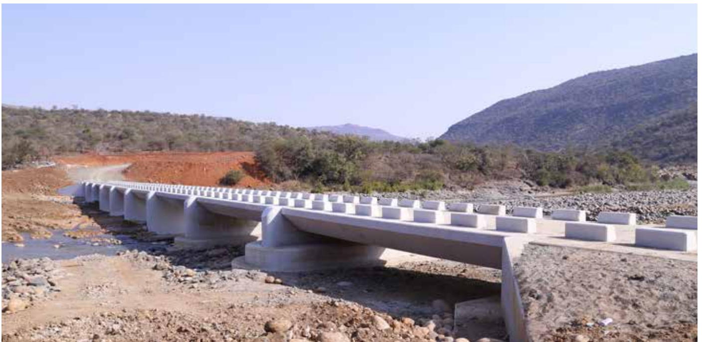
Buffels River Bridge on local road L2953 in the Mahlaba area in Msinga Local Municipality. This bridge connects Msinga to Nquthu.
